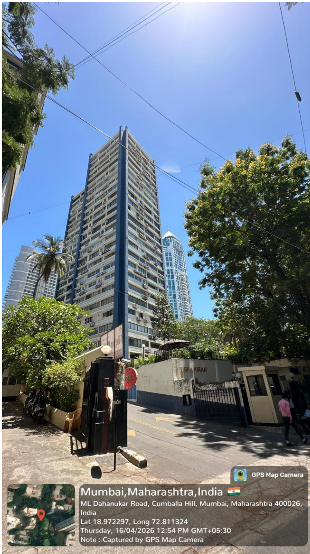
Image 1: Flat in Usha Kiran Building on M.L. Dhanukar Road, Mumbai, Maharashtra registered in the name of Mr. Anil D. Ambani.
